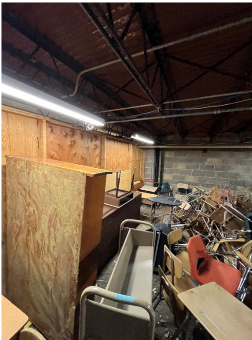
Photo #TC7 – Basement storage room
