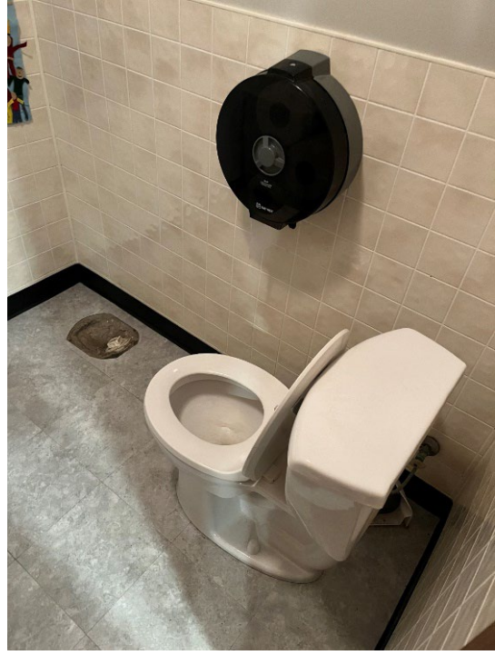
Photos – #HF10– Uncovered opening and toilet location
